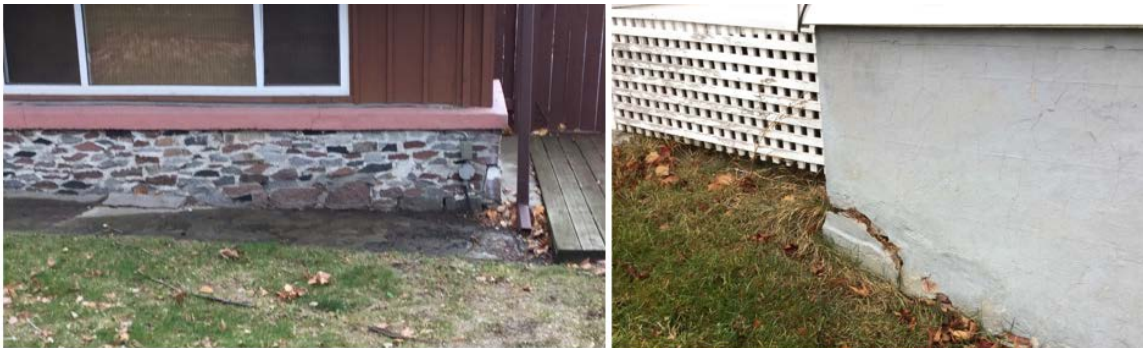
Figure 7: Examples of Damaged Foundations
